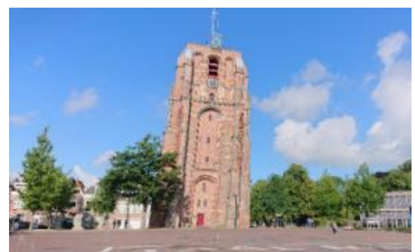
The unfinished leaning Oldehove tower
