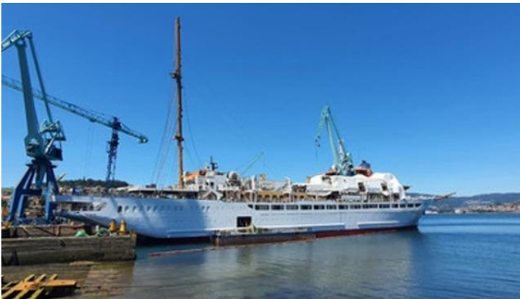
First mast in position on the Sea Cloud Spirit – photo courtesy Sea Cloud Cruises
